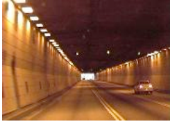
Figure 1: Un tunnel routier.
